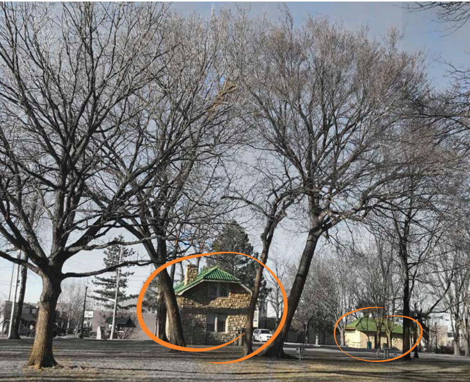
Structures on site.
